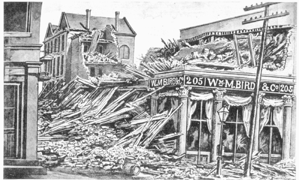
EAST BAY, CORNER OF CUMBERLAND STREET—A COMPLETE WRECK Damaged $15,000.
